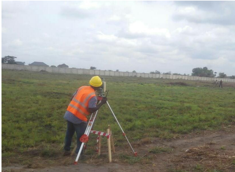
Setting out of building using a total station instrument
