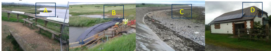
A) Panoramic view and signs in the Lake, B) Repairs of the inlet, C) Litter on the external side of the barrier, D) The House
