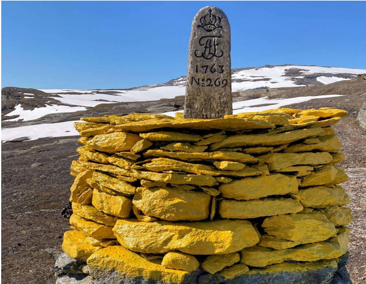
Figure 1: The main part of those boundary markers that were erected during the 18th century consists of about 1.5 metres high stone cairns with flat stones with engraved royal monograms. The Swedish side bear the monogram of King Adolf Fredrik, as here on boundary marker no 269.
