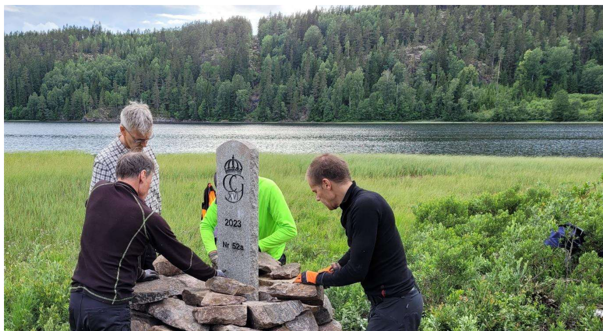
Figure 8: One new boundary marker that defines the boundary has been erected during the review of the boundary 2020–2024. The work with building the cairn was performed through joint efforts by Tor Erik Bakke, Anders Østeraas, Martin Lidberg and Dan Norin from both boundary commissions. The boundary marker is designated 52a and the location is in a break point that so far only has been defined in earlier maps. Boundary marker no 52 is visible on the other side of the lake in the boundary clearing.
