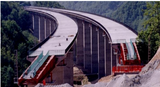
Figure14. ILM Construction Method
