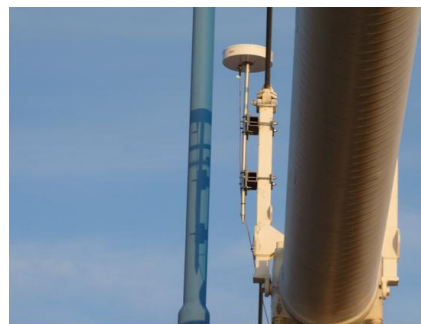
Figure 5. GNSS choke ring antenna located on the suspension cable.
