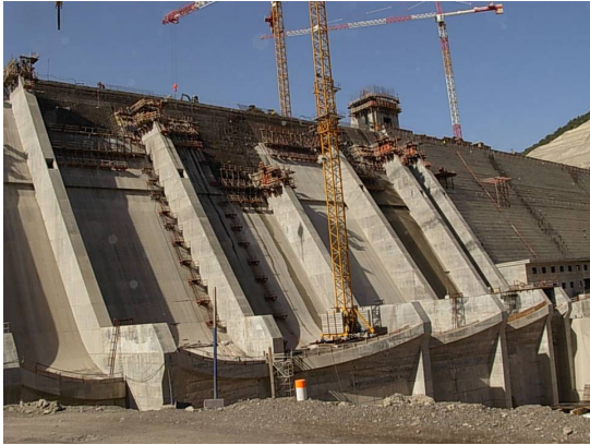
Figure 9 – The Koudiat Acerdoune dam under construction
