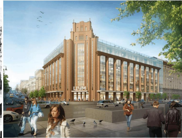
Fig. 2 Exterior view of the facade after reconstruction in 2016
