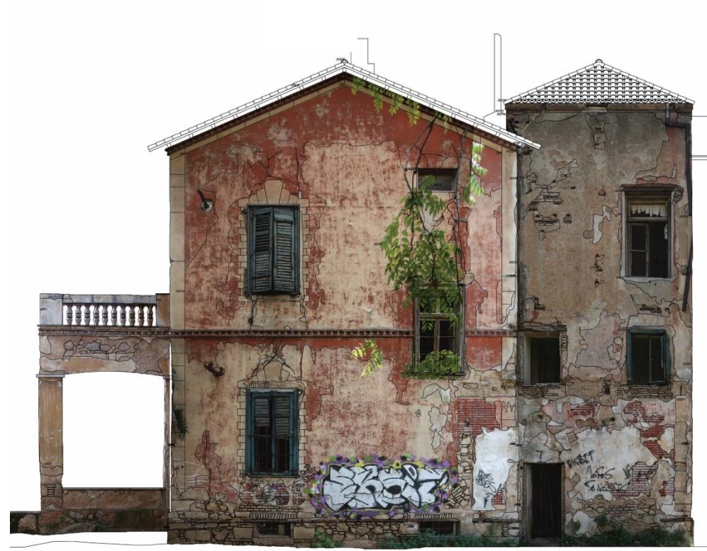
Lab of Photogrammetry, Orthoimage of the North Facade
