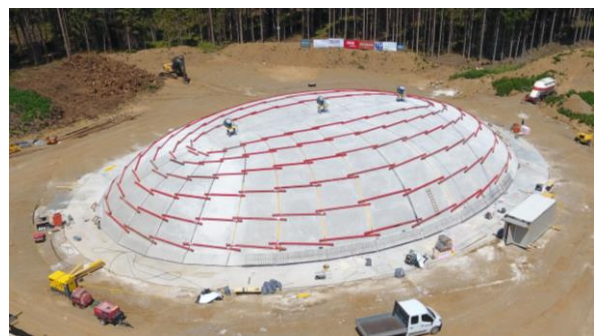
Figure 1: Wildbrücke after the lifting process with iron beams minimizing the shear stress
