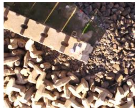
Figure 7 – Surface of a breakwater with an accessible area (painted orange points are perceivable) surrounded by an area covered with rock and Dolos blocks (these ones at the bottom of the photo)
