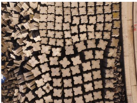
Figure 8 – Aerial photograph of a breakwater made of Antifer blocks, regularly placed
