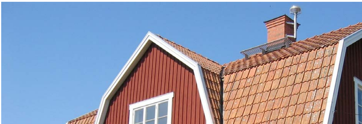
Figure 2-2: Söderboda is a SWEPOS station with a roof-mounted GNSS antenna mainly established for network RTK purposes belonging to Class B.
