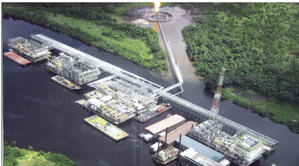
Fig. 2: Photo Showing the North Water Station of Study Area
