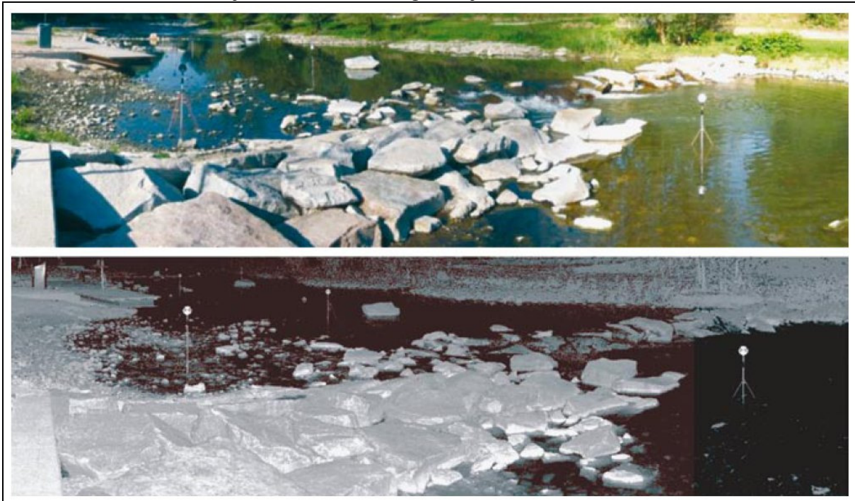
Figure 2: Photograph (above) and TLS point cloud (below) show a stone sill in the project area
