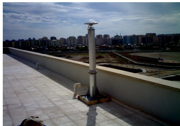
Figure 3. Galvanized steel pillar (3 m)
