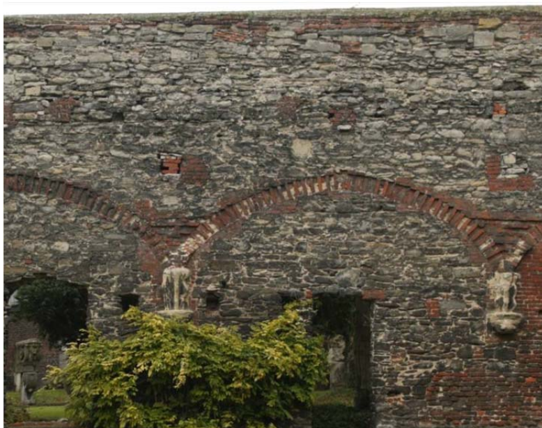
Figure 4: Sint-Baafs Abbey – Orthophoto of a part of the wall (2010)
