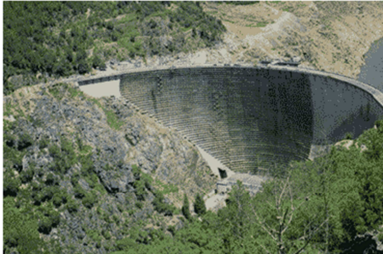
Figure 13 – Repair works in Cabril dam
