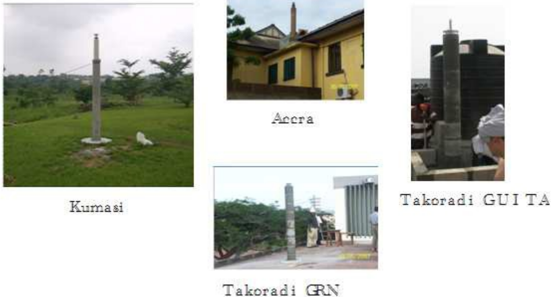
Figure 1.1: Monuments for the Permanent Stations
