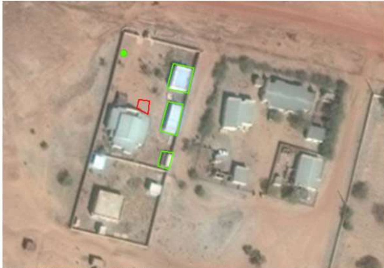
Reconstruction of a public health center in Dauteriv, Mali. Photo: UNDP
