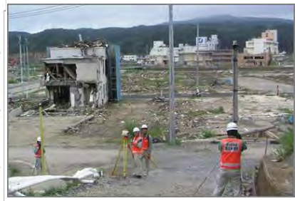
Leveling after 2011 Tohoku EQ
