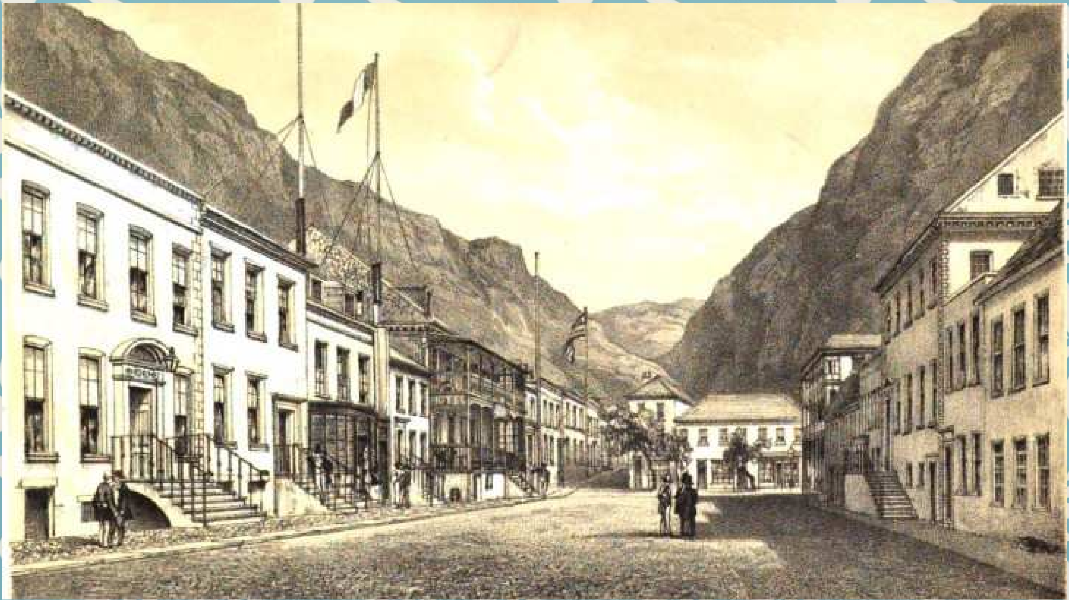
SLIDE II – A VIEW OF THE UPPER PART OF MAIN STREET, JAMES TOWN
